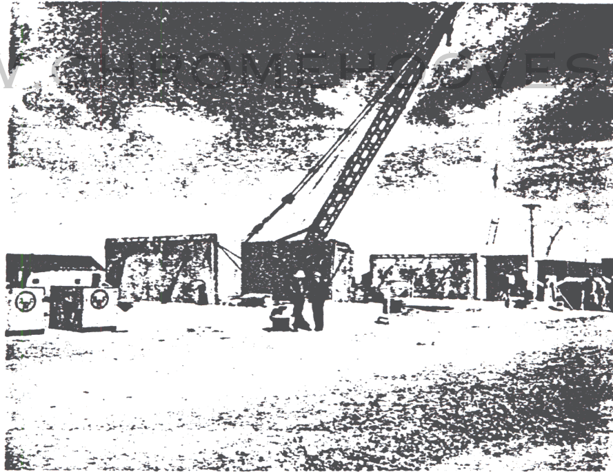
TYPICAL VIEW OF ANTENNA SILO AREA WITH SILO DOORS OPEN
