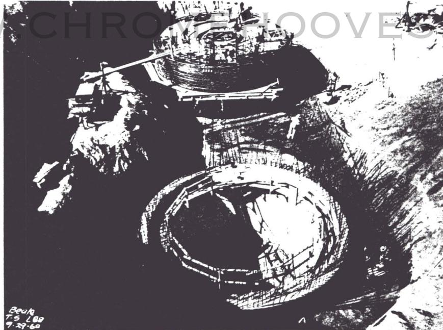
Compacting Backfill Antenna Silos, Site 1A Fig. 29
