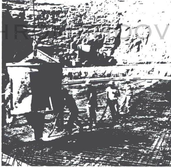
Concrete Placement Showing Concrete Buckets, Site 1A
